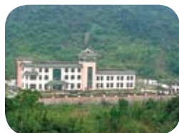
A WATER INTAKE PUMP STATION IN CHINA WHERE CASCAL MANAGES WATER SERVICES
